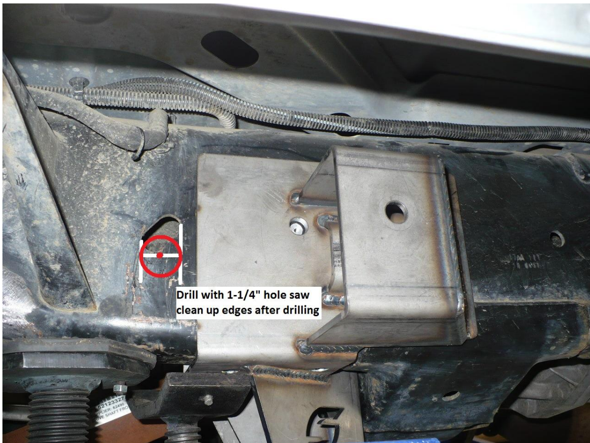
IMG 15.2 Hole saw location to drill for nut tab installation.
